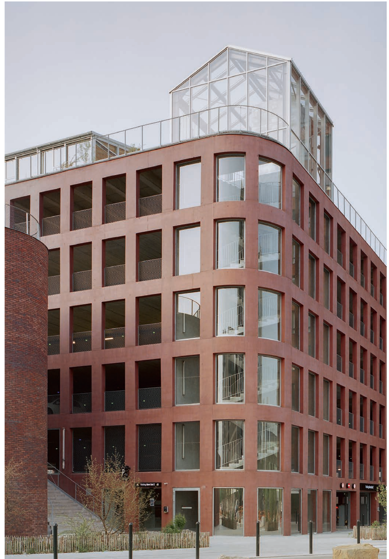
Offices, silo public parking and collective housing, Nantes, France; Architecture: Raum; Luminaire: Scorel
