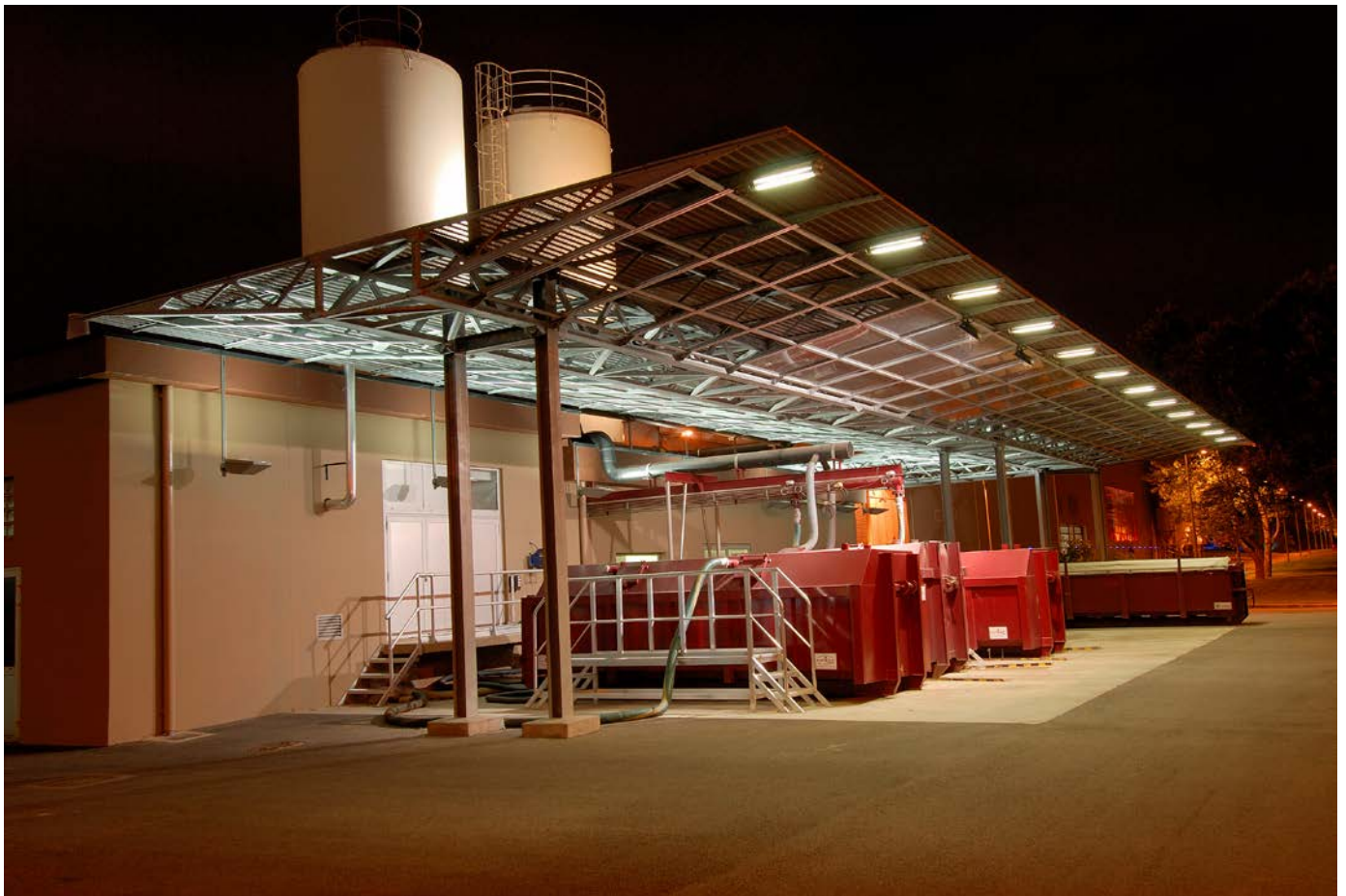
Wastewater treatment plant, Ginestous, France
