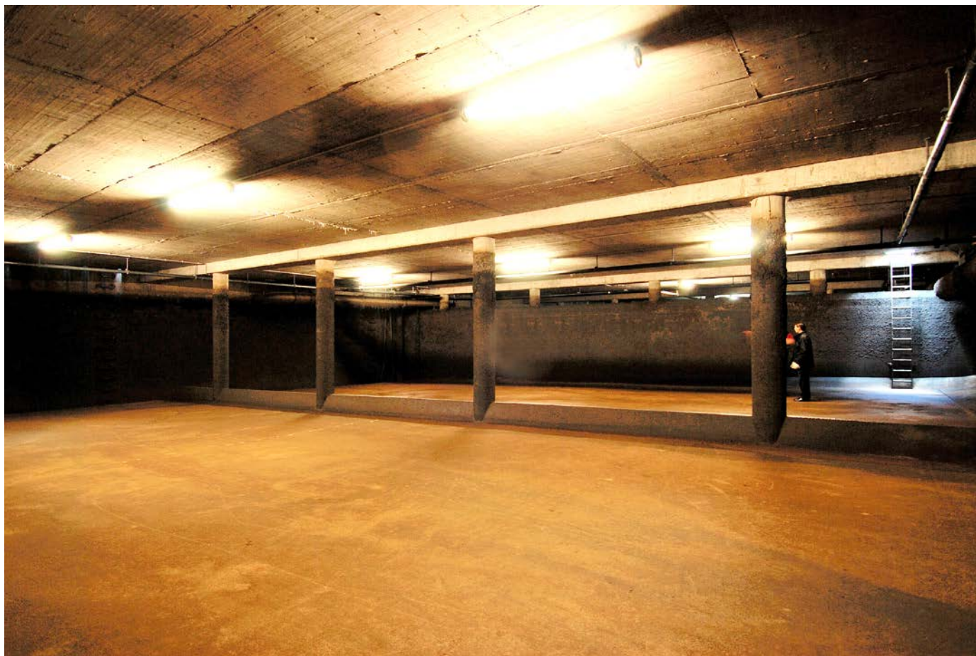
Rainwater recovery basin, Vlotho, Germany
