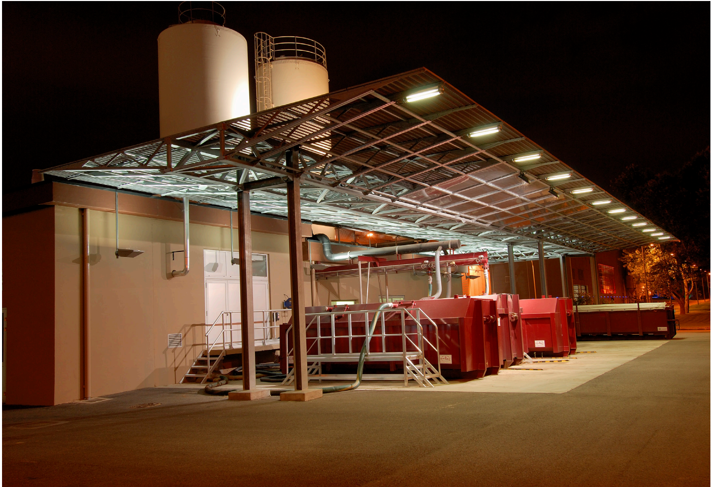
Station d'épuration, Ginestous, France
