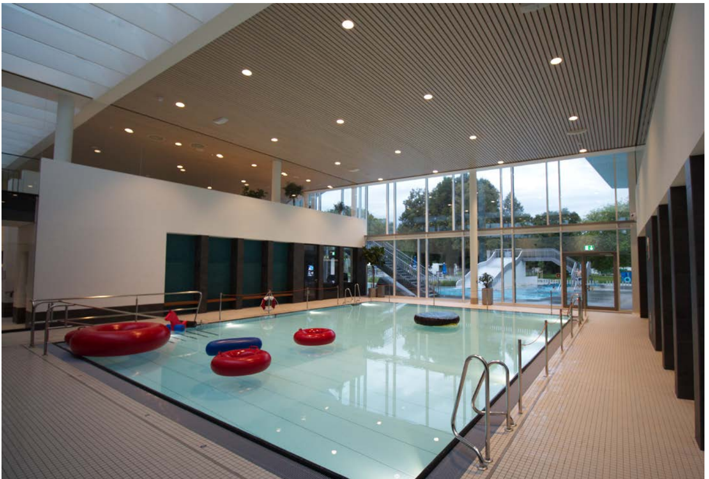
Fresch Swimming pool, Freising, Germany. Architects: Venneberg & Zech. Electrical design: Mr Methling, Ibah ©Michael Schönau; Luminaire: complx. 200
