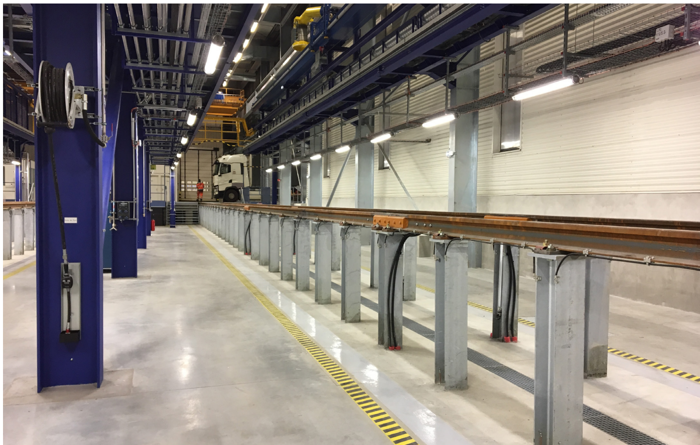
SNCF workshops, France
