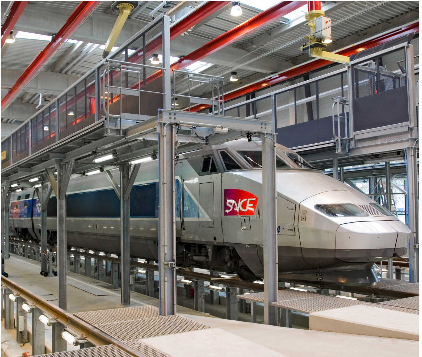
SNCF workshops, France
