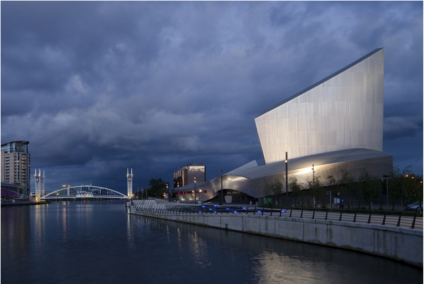
Imperial War Museum North, Stretford, United Kingdom. Luminaire: SILL - 49. Architects: Daniel Libeskind. Light planning: DHA Design ©Hoffmeister
