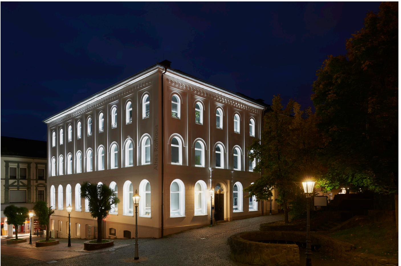
Old town hall, Lüdenscheid, Germany. Luminaire: Hoffmeister - led.modular (special projector) ©Hoffmeister
