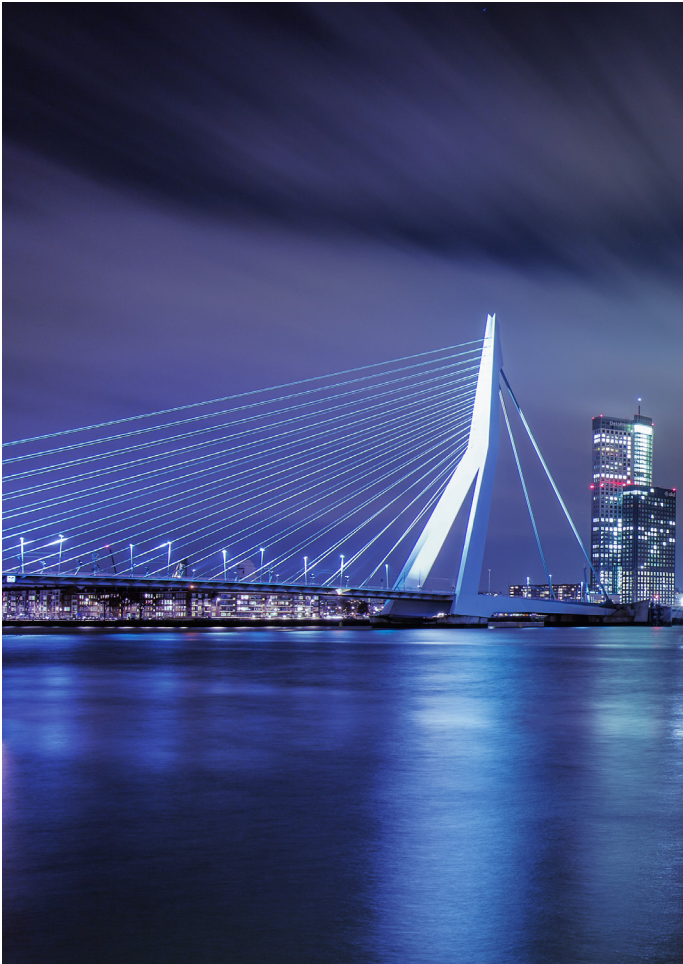
Erasmus Bridge, Rotterdam, Netherlands. Luminaire: SILL - 14L ©Hoffmeister
