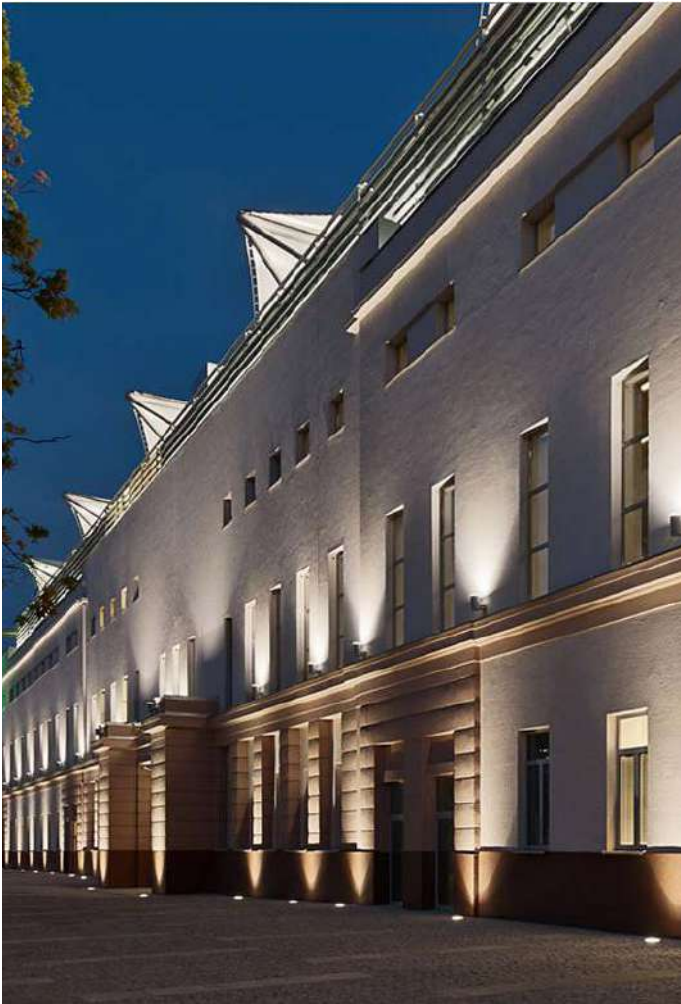
Stadium of Legia, Warsaw, Poland ©Markus Böker; Luminaire: DL 150
