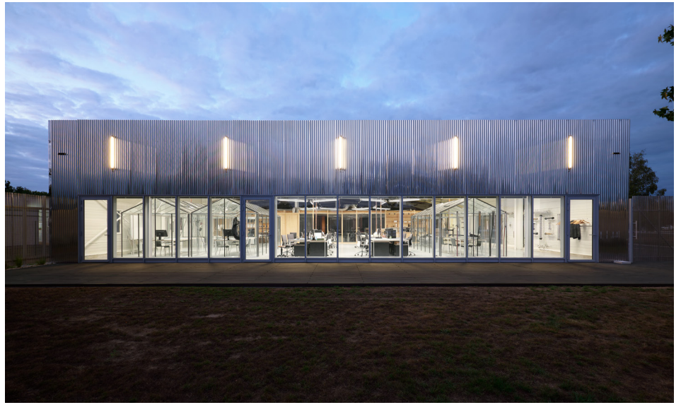
Sammode Research & Development Centre, Lamotte-Beuvron, France
