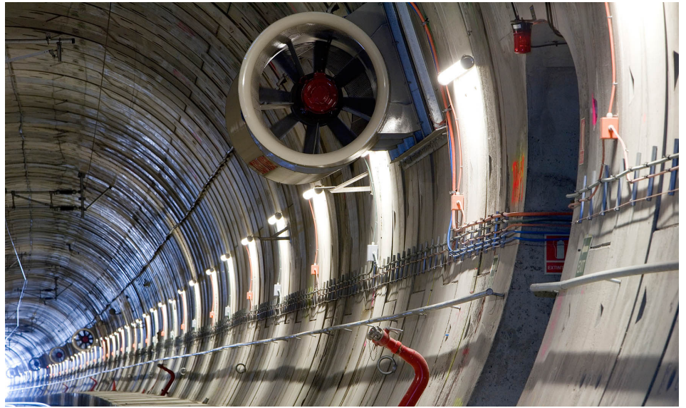
Perthus tunnel, France
