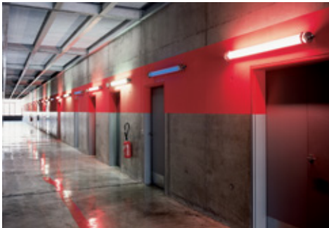
Resin gives a wet look to the concrete floor of a ground-level corridor in the fire station that Ibos-Vitart Architectures built in Nanterre, a Paris suburb.
