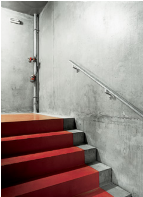
The emergency-exit stairwell's painted steps.
