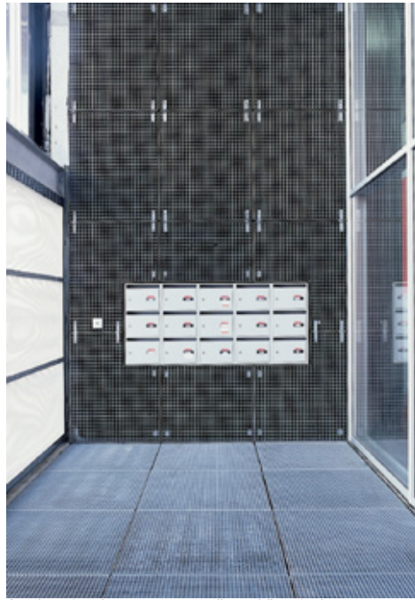
Steel grating that serves as walls and floor in the apartment block's mail room.
