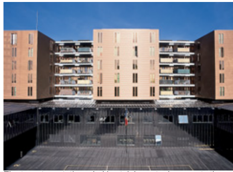
The two-story station, clad in stainless steel, supports the apartment block, clad in copper-tinted aluminum.
